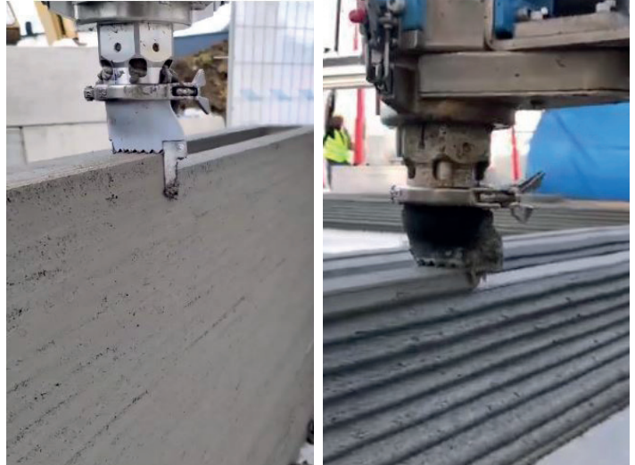
Fig 31. Print using two layered flap Fig 32. Print without flaps
